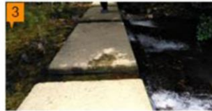
Description of Existing Condition during visit
